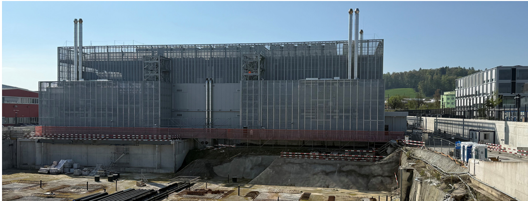
"Hyperscale location" ZRH2 of Green Data Center in Dielsdorf (Image: courtesy of the publisher)
