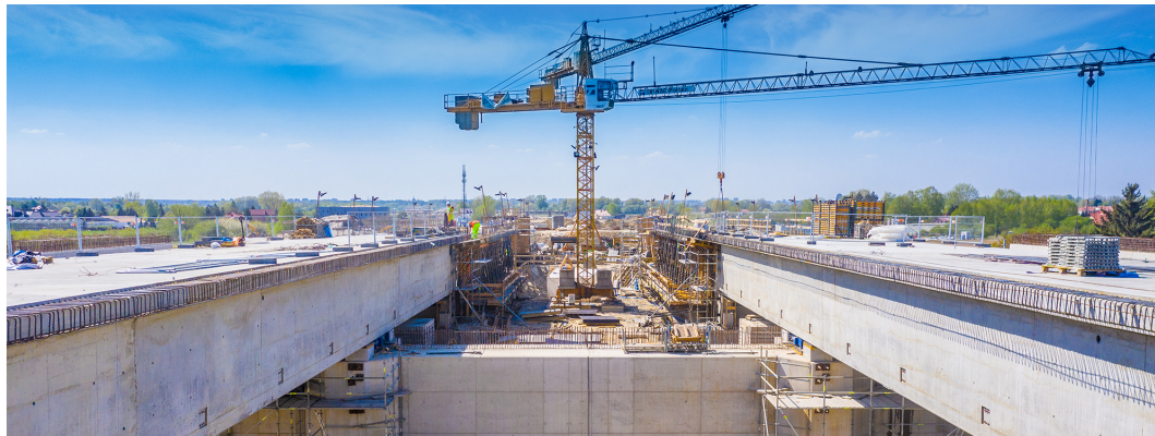
Expansion of transport infrastructure (image source: stock.adobe.com)
