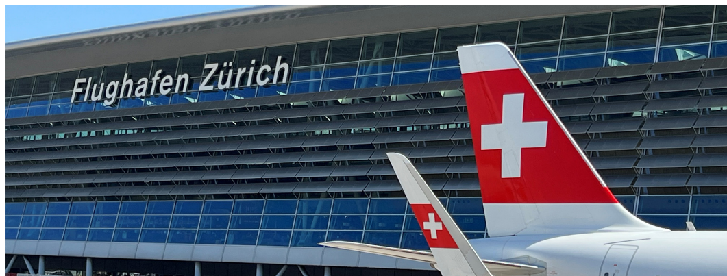
Transport infrastructure is central to a prosperous economy (Photo: Maurice Pedergnana)
