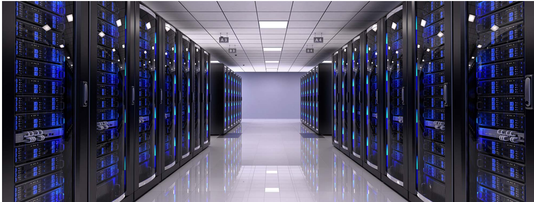
Modern Data Center (Image source: stock.adobe.com)
